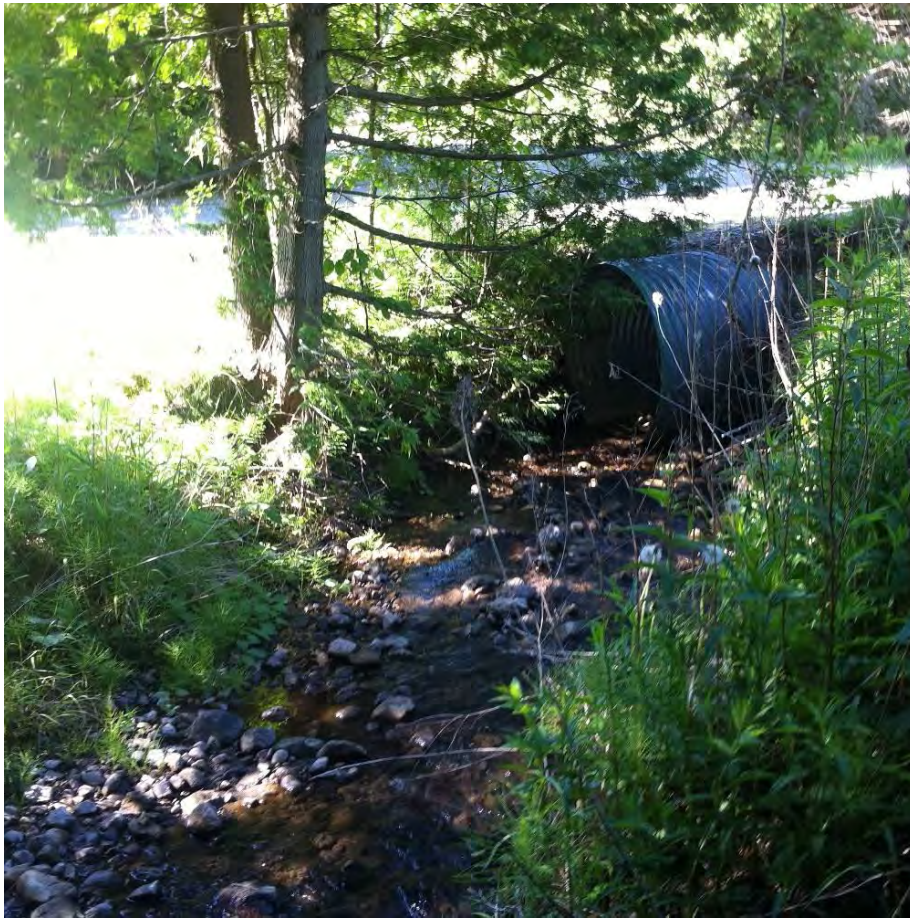
Figure 6 – 1.2m Driveway Culvert off of Hutsell Road
