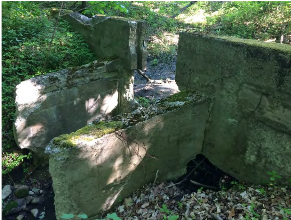
Figure 2 - 1.2m Wide x ~1.5m Tall Weir Structure - Inline
