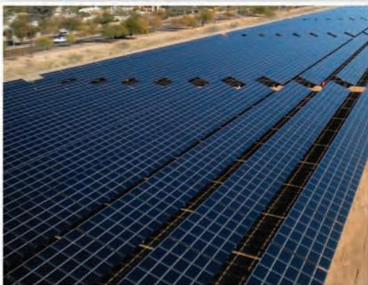
The Solar FlexRack can accommodate solar modules in both portrait and landscape orientation. Installation is fast and easy, and the Solar Flex Rack's unique power-grab clip facilitates the installation of heavy modules. When you combine this with the installation speed of the Solar FlexRack itself, you can greatly reduce your balance of system cost by using the Solar FlexRack.
