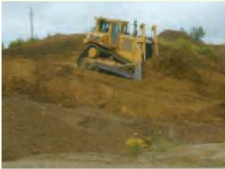
Dozer pushing soil from boundary berm
